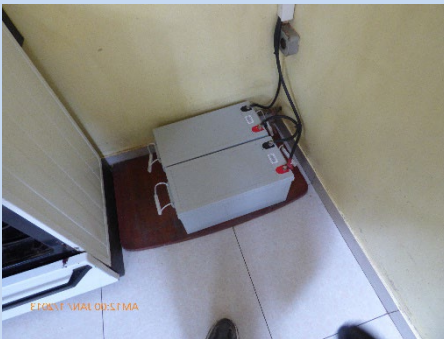
New solar electric system batteries
